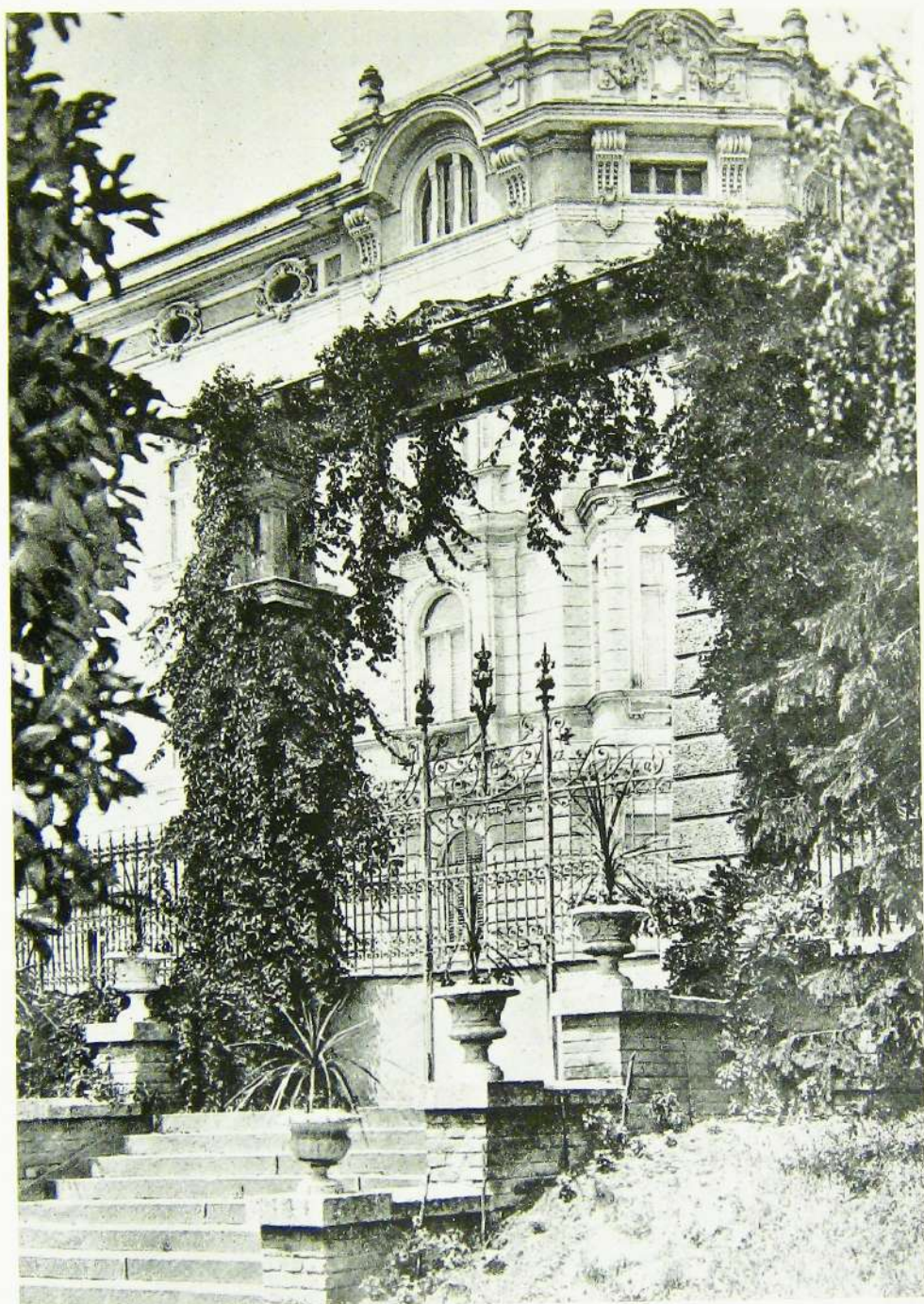
Glavni ulaz 1920.g. Haupteingang um 1920. Main entrance around 1920.
