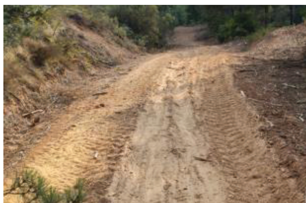
Figure 3. Field measurement points on cross section on skid road
