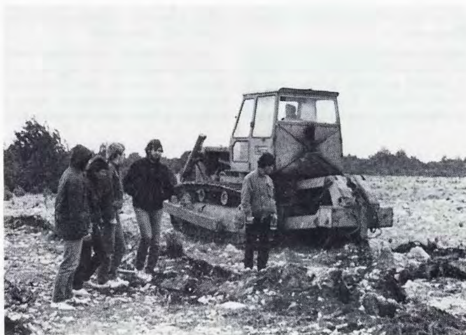
Sl. – Fig. 5. Podrivanje kraškog tla ripperom na području OOUR Šumarije Šibenik, Šumski predjel Lozovac-Gulini (Studentska terenska nastava, travanj 1985. god.) – Undermining of karst soil by rippers in the Šibenik forest management, the Lozovac-Gulini forest area (Students' practical studies, April 1985)
